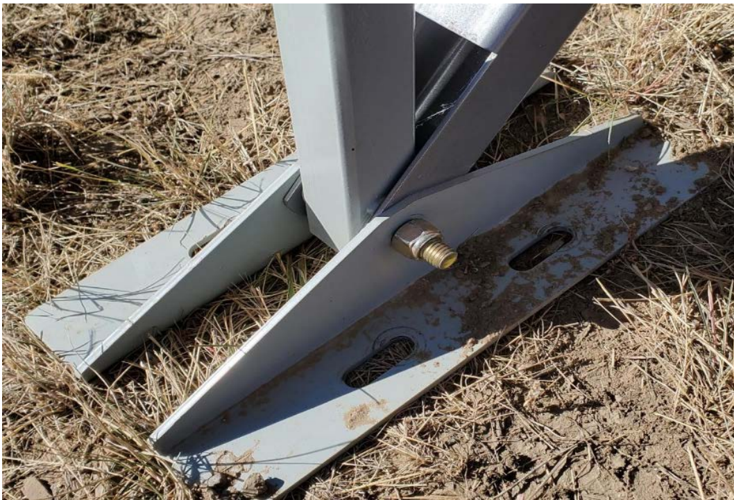
Figure 8: Close up of Legs
