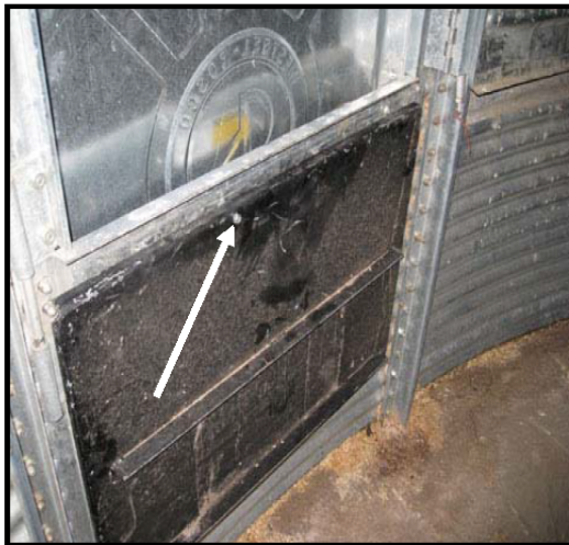
Attach with 3/8 x 2" bolt and nut enclosed
