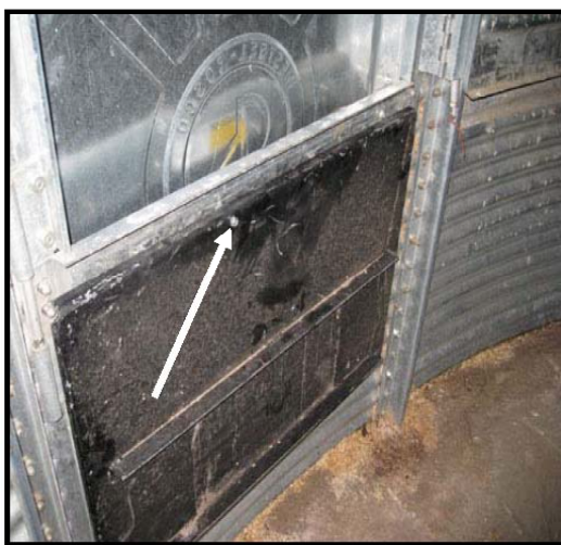
Attach with 3/8 x 2" bolt and nut enclosed
