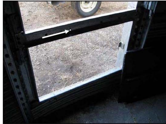
Open bolt hole in center bar
